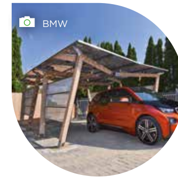
BMW Solar Carport South Africa
