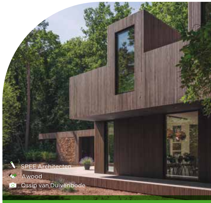
SPEE House outdoor beams installed on façade and sloping roof with Grad system - (10.000 m) The Netherlands
