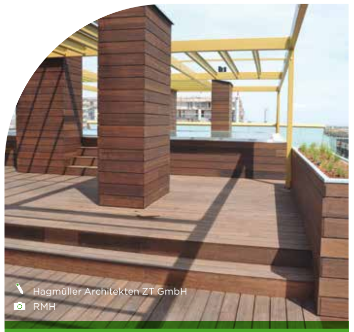
Residential building Braunhubergasse 28 (1580 m 2 ) Vienna, Austria
